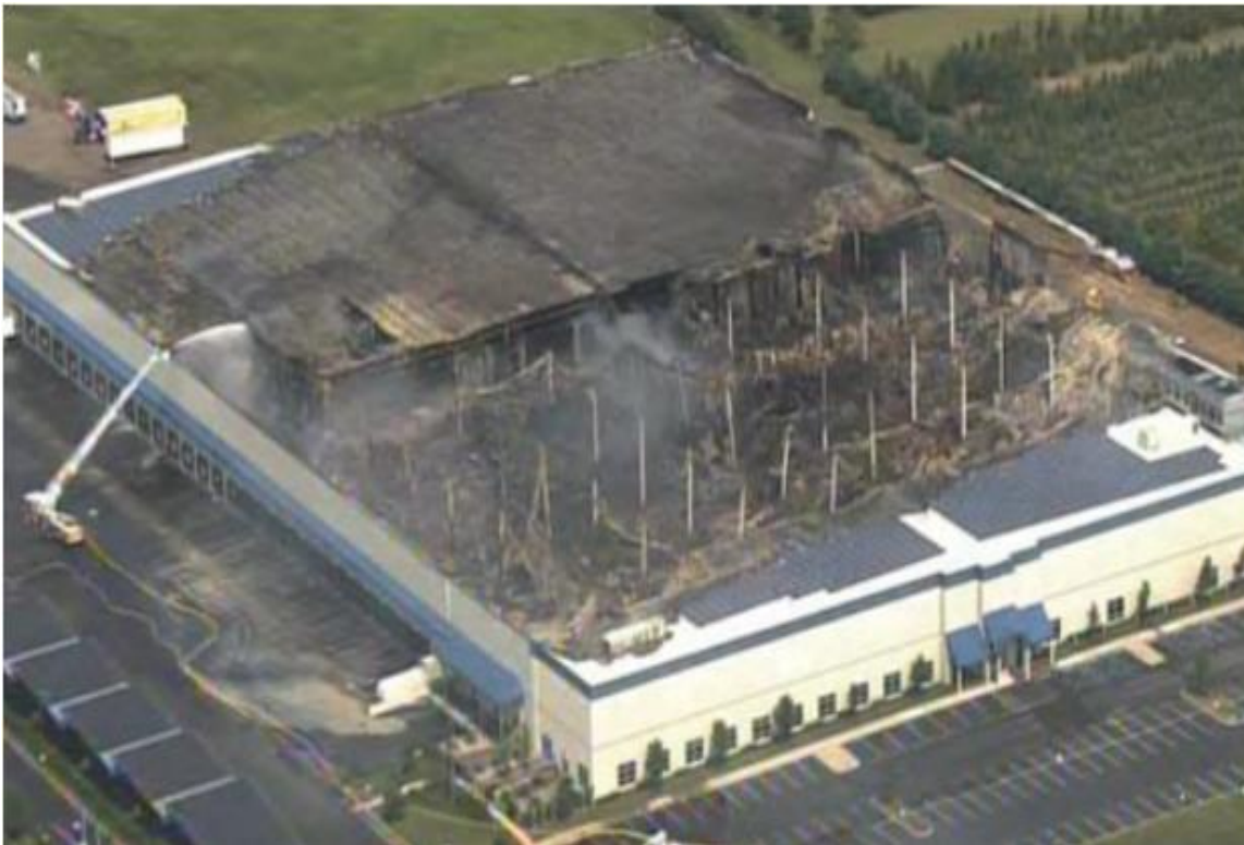
Delanco, New Jersey, US in September 2013: a fire occurred at a cold-storage food warehouse that was approximately 300,000 ft 2 (28,000 m 2 ) in size with more than 7,000 PV modules covering most of the roof.
